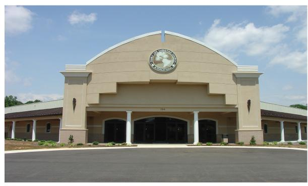
Construction of a modern, new 24,000 square foot church with 750-seat sanctuary, classroom, office and daycare space, as well as audio/visual control areas and lighting to televise the services. This is a pre-engineered building with EIFS and masonry veneer. The project was developed and constructed on a "team" build basis with the architect, owner, and C.L. Lewis & Co., Inc.
